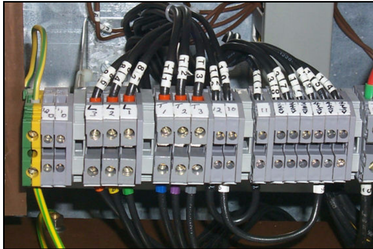
Figure. 7.12 9PSU Single Phase Terminal Block Link
