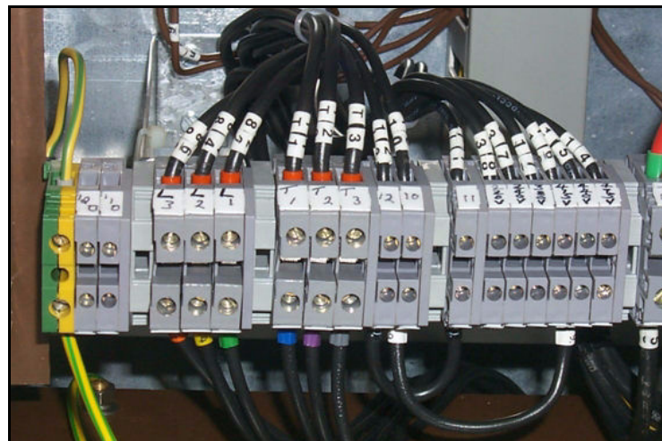
Figure. 3.2 9PSU Terminal Block
